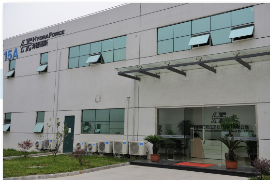
PRECISION MACHINING AND MANIFOLD ASSEMBLY FACILITY IN CHANGZHOU, CHINA, NEAR SHANGHAI
