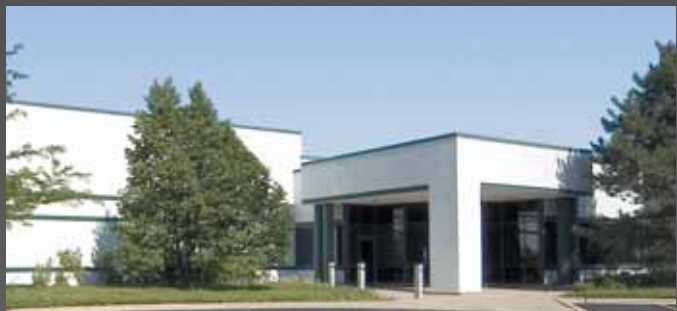
Precision machining facility in Lincolnshire, Illinois.
